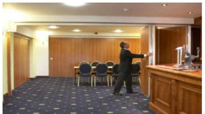
Figure2: wooden folded partitionable system, source: www.buildingaddition.co.uk multifold, [12]. (2016).
